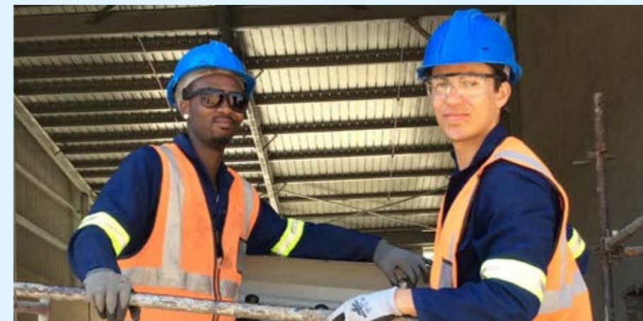
Two proud apprentices at work are Sonwabile Mzaydume and Moegamat Isaacs from Graham Clarke Electrical
